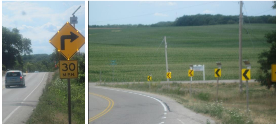
Figure 3-1 TAPCO Curve Warning and Chevron Signs
